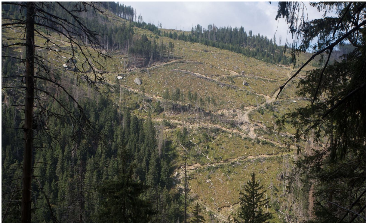
Fig. 15 New roads on steep slopes cause erosion and changes in hydrological regime.
