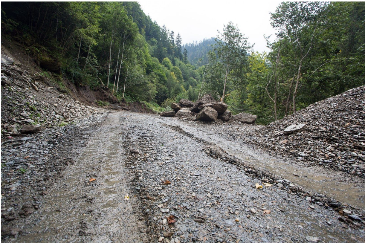
Fig. 3 A huge forest road has been rebuilt into the valley.
